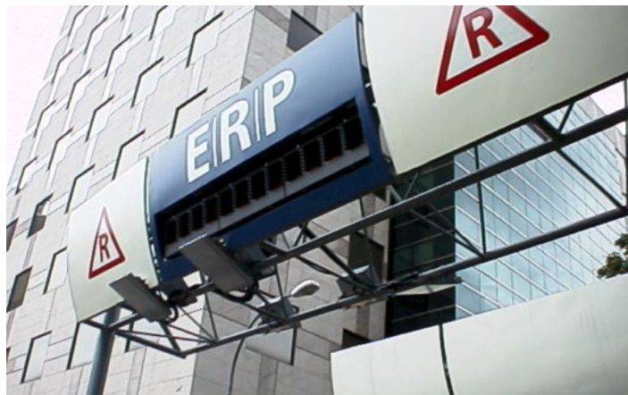
Figure 1: Automatic tolling gantry of Singapore's Electronic Road Pricing system
